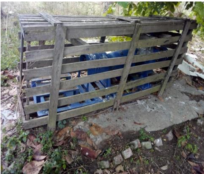
Packed new disposal pump lying in open place but not installed (para 4.3.1)
